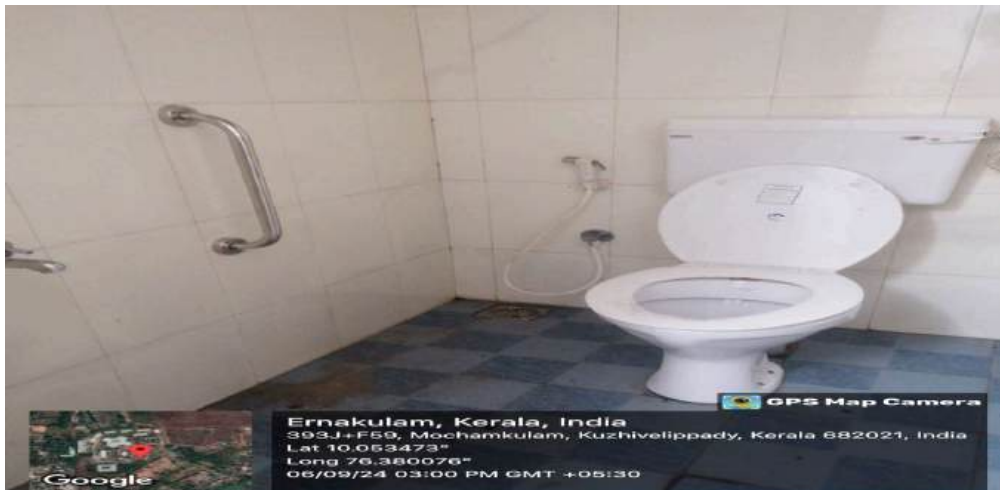
Divyangen Friendly Toilet
