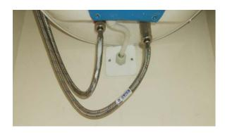
The 7X7cm glanded plate cover is made high quality black-steel plate enameled with primer and RAL9016 Crème color electrostatic painting. The cover plate comprises two horizontal oval opening for fixing screws. The oval shaped openings provide some maneuvering that makes installing easier and faster.
