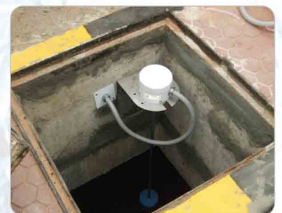
Mounting inside septic tank access using stainless steel right-angle-bracket.
